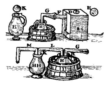
A. Signifies the ash hole which must be as wide as the furnace and always open that the fire may burn the stronger. B The middle hole of the furnace for the putting in of coals.
